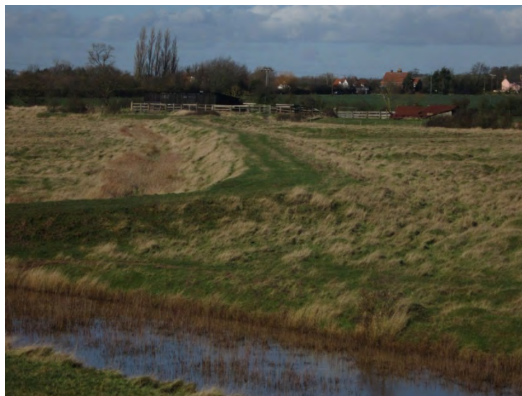
Fig. 7 Raised causeway across Langenhoe Marsh, Colchester
