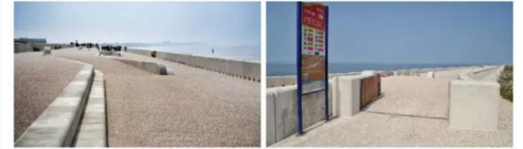
Celebrations as £63m coastal flood defence project is opened
